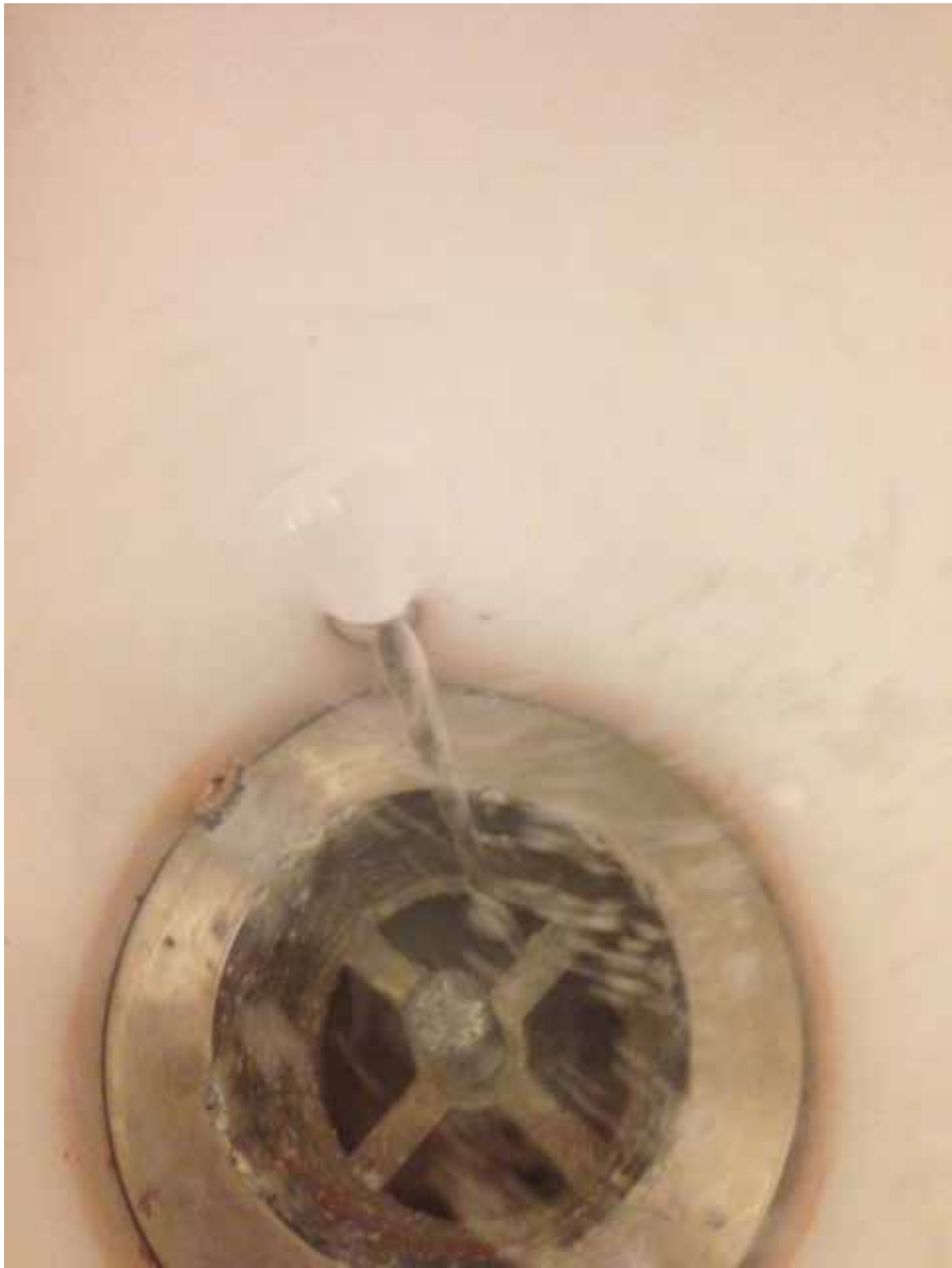
"I had my eyes closed and could hear the drain quickly draining water. I took the photo right before all the water ran out."
